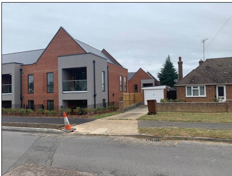
Figure 4: Relationship between East Stour Court and 21 Mabledon Avenue.
