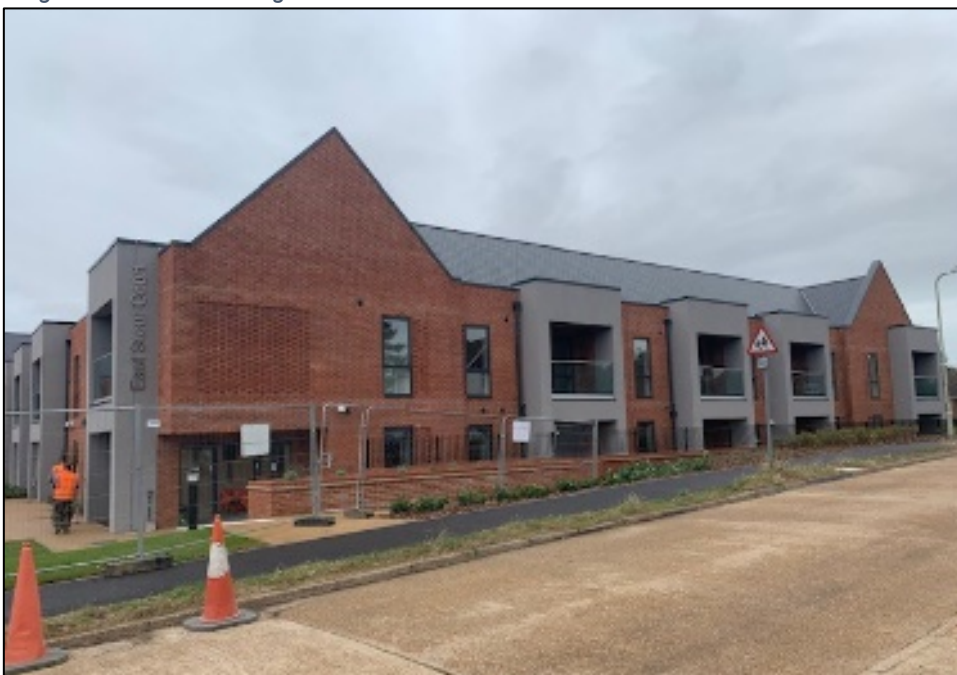
Figure 3: Continued Front elevation of East Stour Court facing onto Mabledon Avenue.
